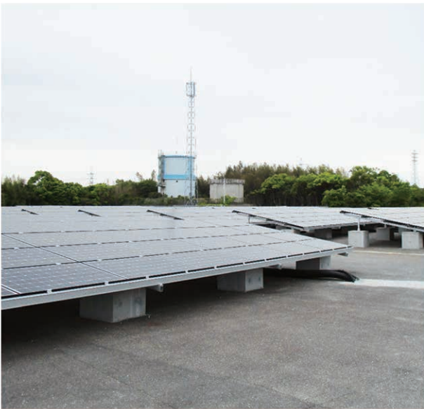
Solar power generation facility
