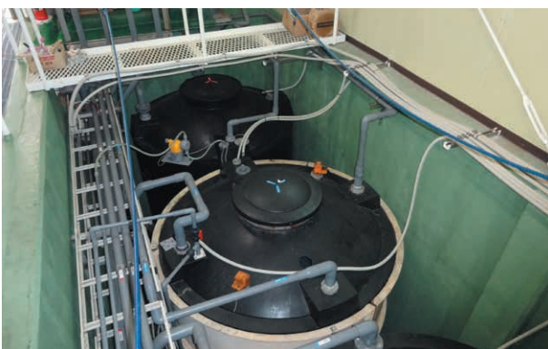
Waste liquid tank
