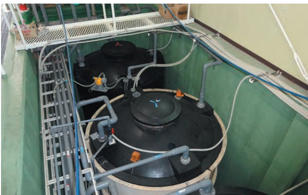
Waste liquid tank
